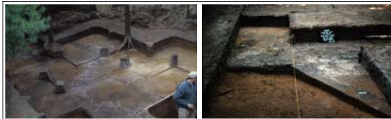
Overview photo of site excavations
