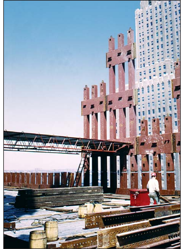
Figure 2-8 Erection of floor framing during original construction.
