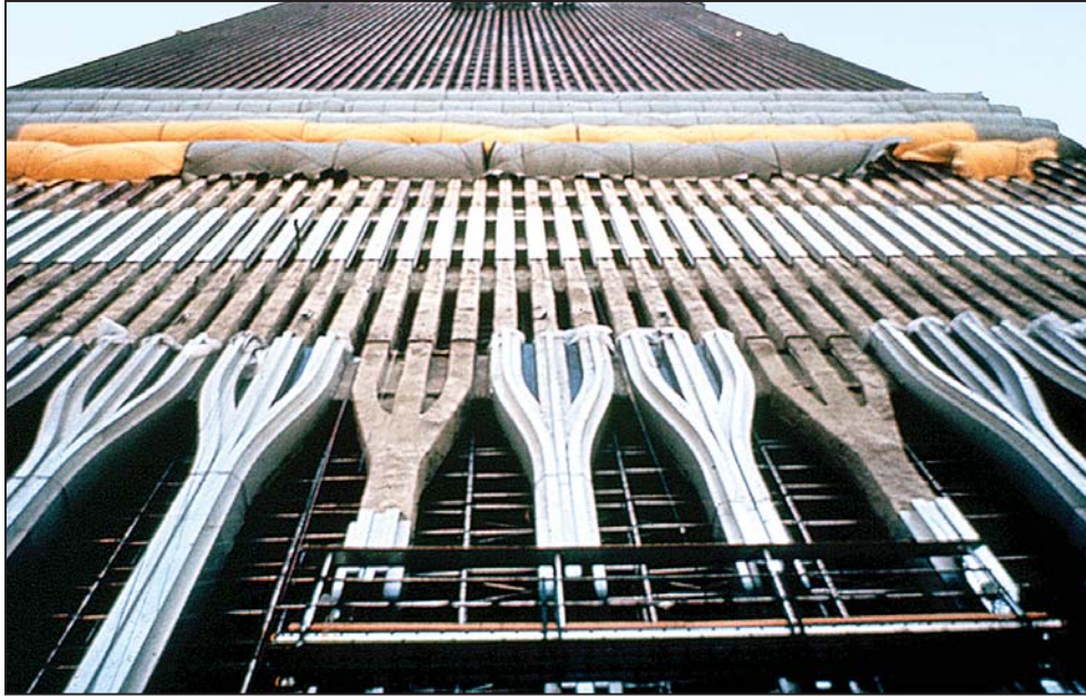
Figure 2-4 Base of exterior wall frame.
