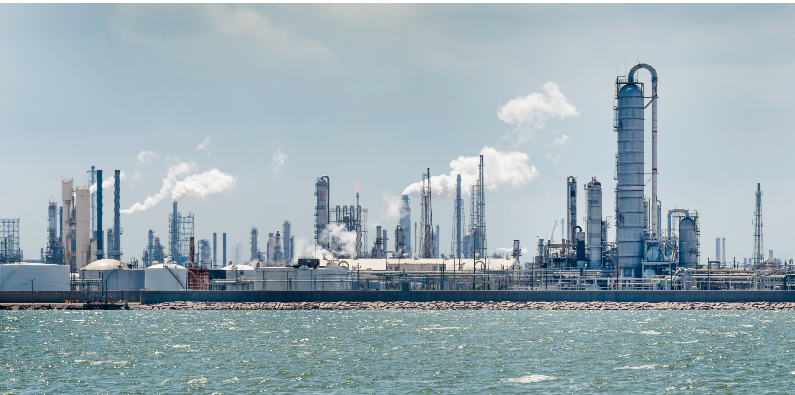
Petrochemical processing plant, Texas City, Texas. ©istockphoto
