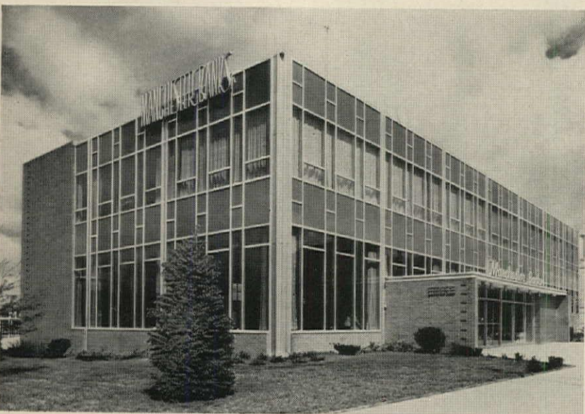
Manchester Savings Bank, Manchester, N. H. Architect: W. G. Knoebel, AIA, St. Louis, Missouri—Associate, John D. Betley, AIA, Manchester, New Hampshire Consultant & Contractor: Bank Building & Equipment Corporation of America, St. Louis, Mo.
