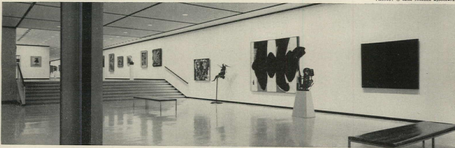
Ten-foot plaster grid covers gallery beneath auditorium, incorporating wiring, air supply, and partition tracks in neat 2-inch slots.
