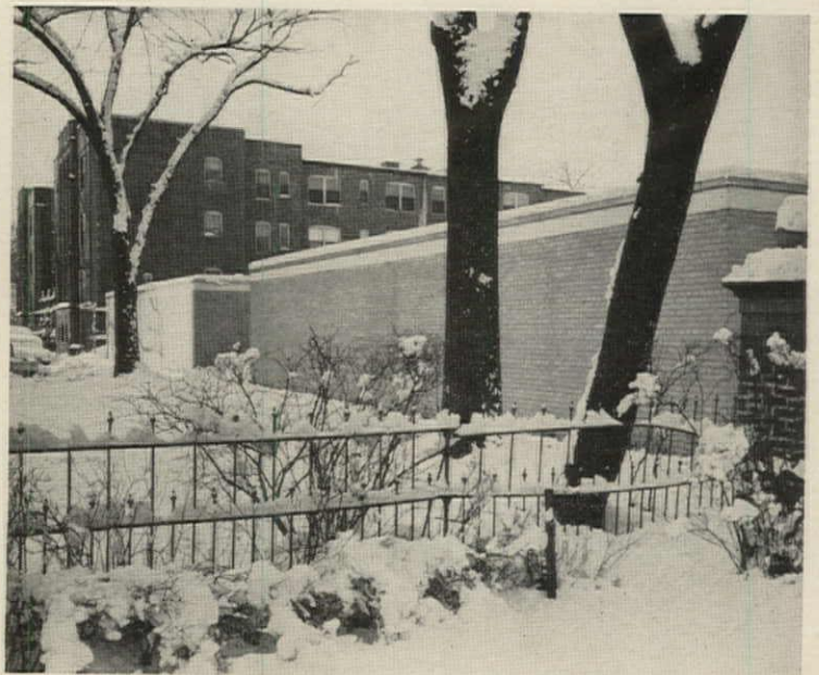
Toward the street and other back yards, the low walls have no openings
