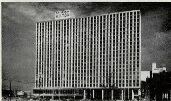
Pittsburgh Hilton, Pittsburgh William B. Tabler, Architect, New York Turner Construction Co., Gen. Contractor, Philadelphia Hardware Engineers & Contractors, Builders' Hardware Contractor, Greensburg, Pa.
