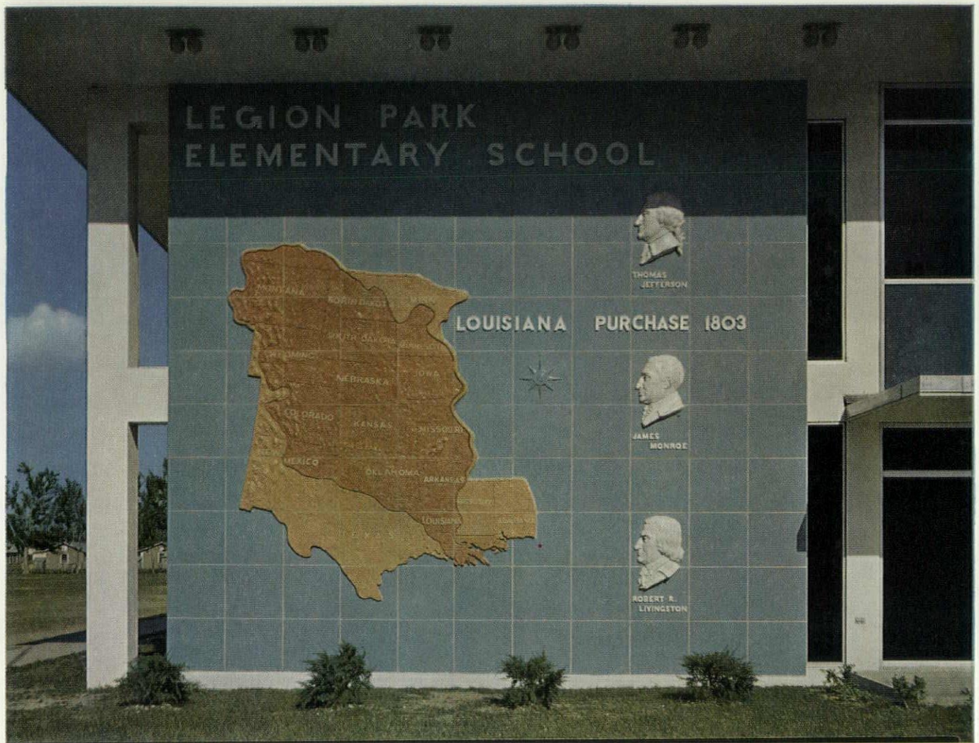
LEGION PARK ELEMENTARY SCHOOL, HOUMA, LOUISIANA. Fernand Picou—Architect. J. B. Talley & Co.—Builder. Students are reminded of the statesmen and land area involved in the Louisiana Purchase by the Ceramic Veneer polychrome map mural 23½' wide x 21'9" high. Unit size of Ceramic Veneer is 23¼" x 25¼".
