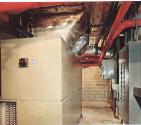
C. Quiet, vibration-free Westinghouse air handling equipment gives the First Methodist church in LaGrange, Georgia, a peaceful, comfortable environment for its congregation. Installation includes Westinghouse-Sturtevant air distributing units, hot-water coils and two 10-ton PB packaged water chillers.
