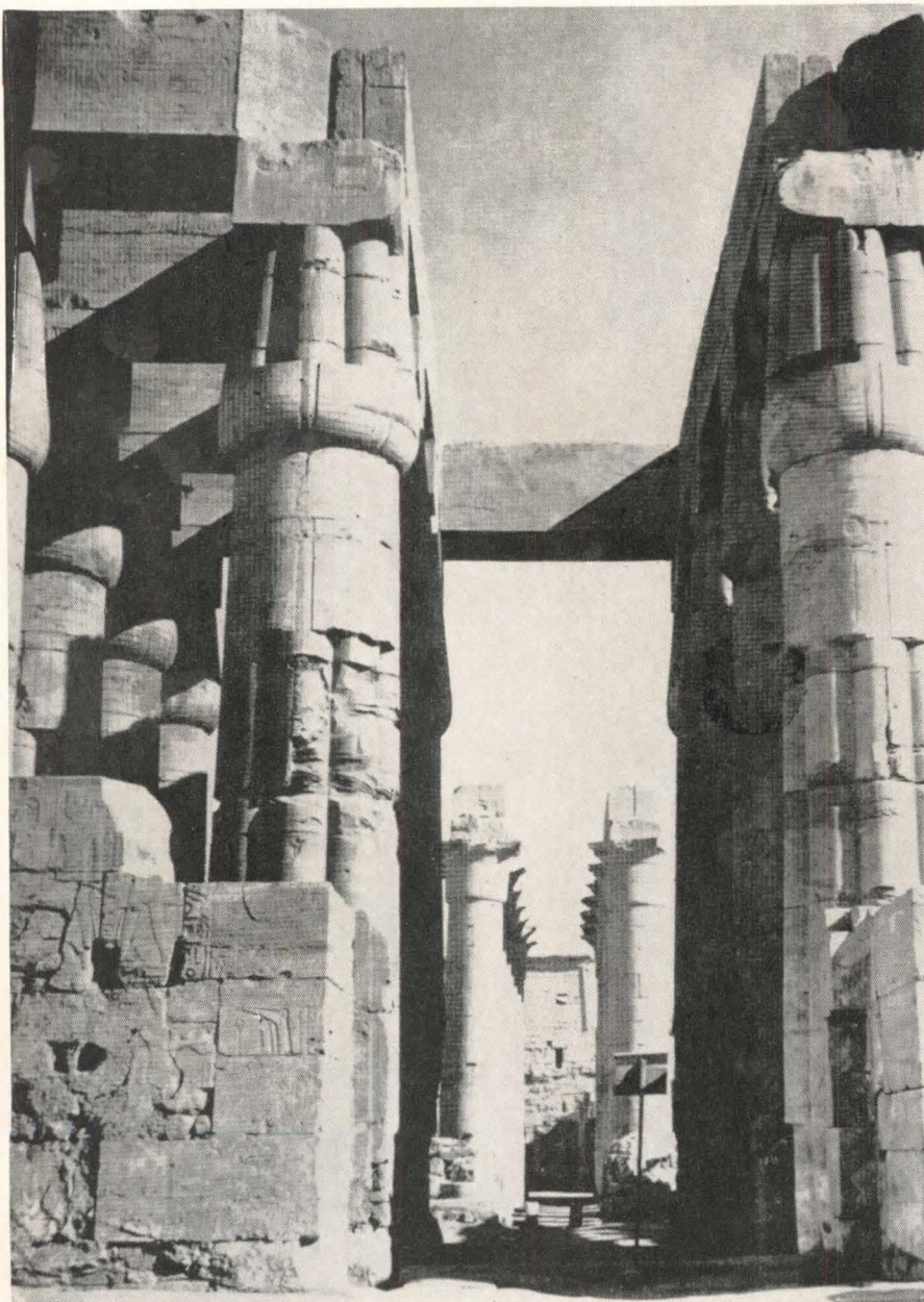
Built at the peak of Egyptian architectural prowess, during the reign of Amenhotep III, the hypostyle hall of the Temple of Luxor demonstrates that "the Egyptians loved half-darkness."
