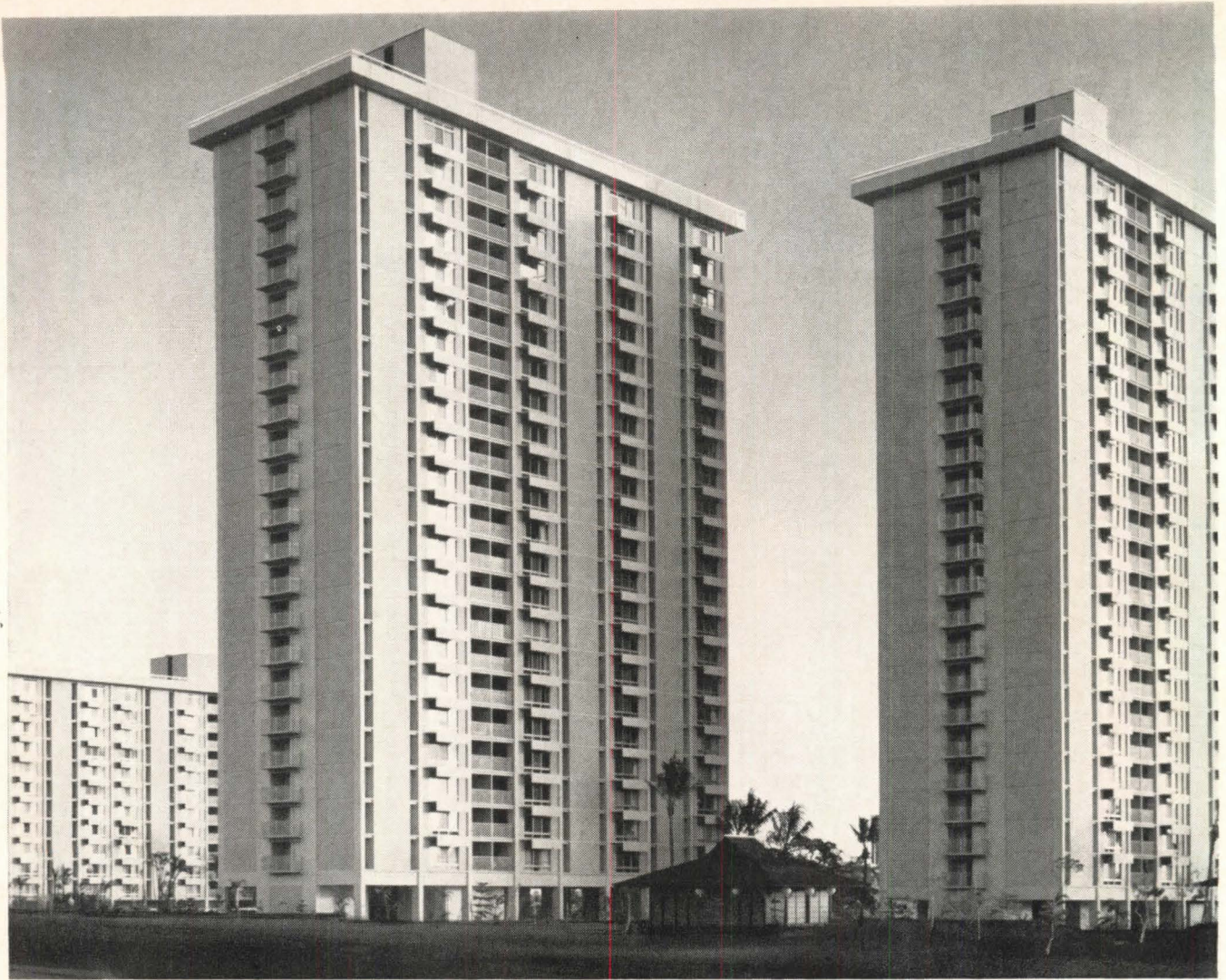
Queen Emma Gardens, Honolulu, Hawaii. Architect and Engineer: Minoru Yamasaki and Associates, Birmingham, Michigan. Contractor: E. E. Black, Ltd., Honolulu.
