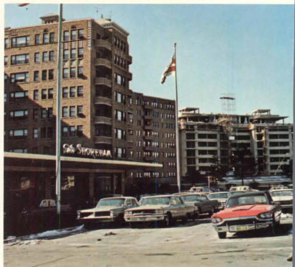
M. Individual-room-controlled air conditioning is used in Shoreham Hotel's new 168-apartment addition. It is supplied by two new Westinghouse centrifugal PE chillers. PEs are smaller, quieter, simpler than any centrifugal equipment now available. Capacities range from 100 to 140 tons.
