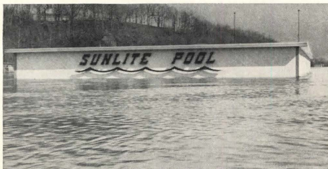
After the flood water receded, the canopy was completely unharmed! Canopy was prefabricated of Ruberoid T/NA 200 and stressed-skin plywood by Batavia Plywood Fabricators, Inc., Batavia, Ohio. The Sunlite Pool is part of Coney Island Amusement Park in Cincinnati.
