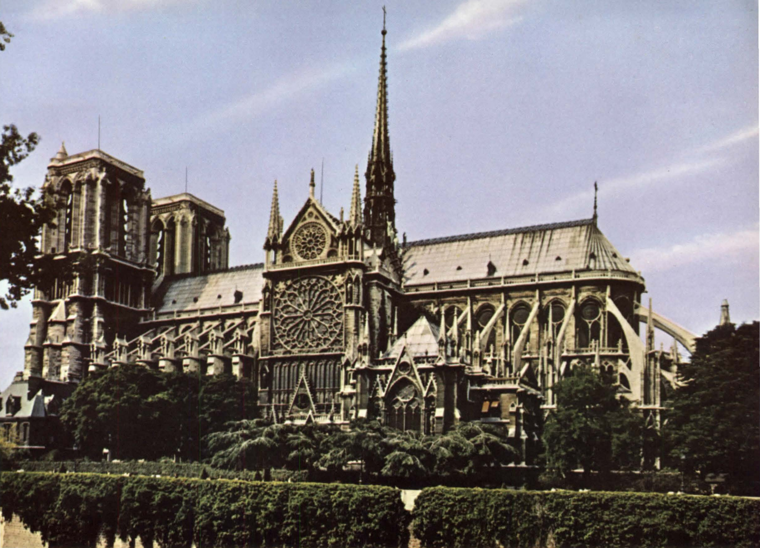
The Cathedral of Notre Dame is the most famous religious edifice in Paris. It measures 139 x 52 yards. Built with very slender internal supports, it exemplifies the grandeur of a balance between vertical and horizontal lines. Central spire was added during 19th Century restoration.
