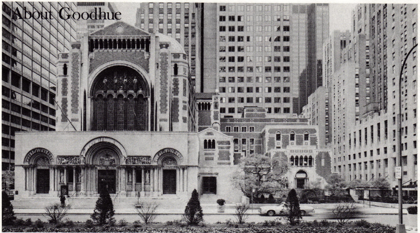
St. Bartholomew's Church, Bertram Goodhue Architect. Photograph by Steve Zone.
