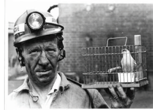
A coal miner holding a canary in a small cage that would warn him about high levels of potentially dangerous gasses.
