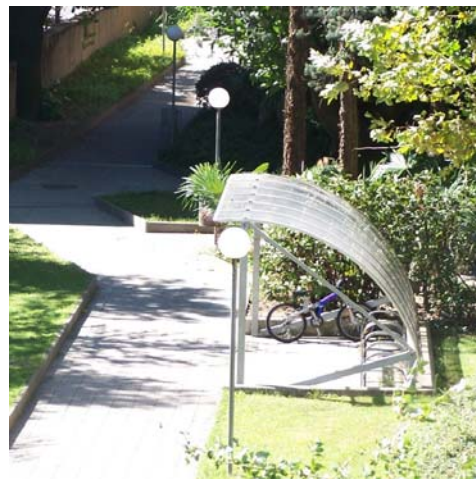
Figure 6: Covered Bicycle Parking
