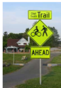
Advance Warning Signs with Subplates
