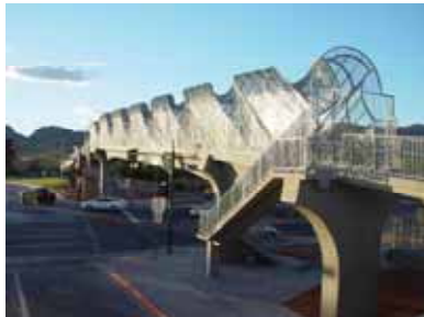
Overpass in Phoenix, AZ
