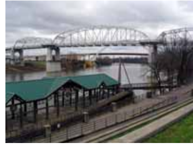
Path Bridge in Nashville, TN
