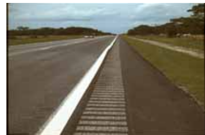
Rumble Strips Placed in the Shoulder of a Highway
