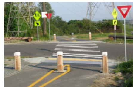
Example Trail-Roadway Crossing with Trail Yield Treatment
