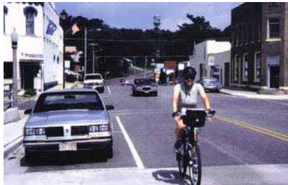
Wide Outside Lane with Parking
