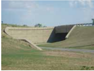
Path Tunnel in Indiana
