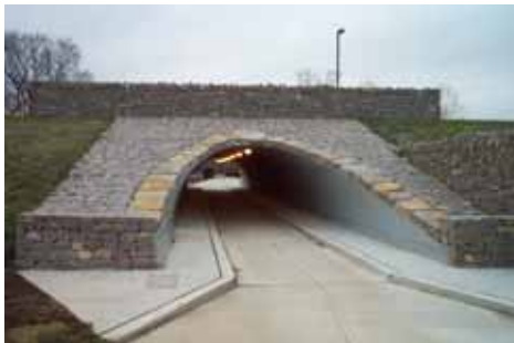
Path Tunnel under Highway
