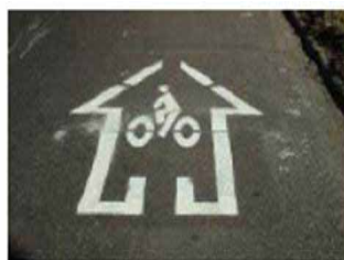
Shared Roadway Pavement Marking in Gainesville, FL
