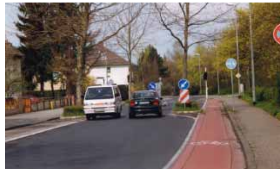
Bike Lane installed at a Chicane
