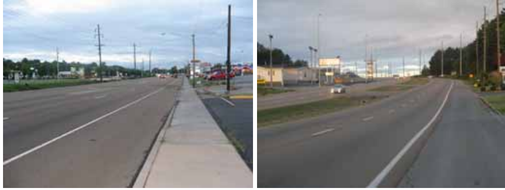
Paved Shoulder on a State Highway in Tennessee
