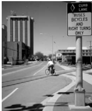
Flared Approach to Railroad Tracks
