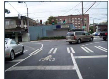
A bicycle box has been installed on N Roy Street to help bicyclists make left turns onto Queen Anne Avenue N.
