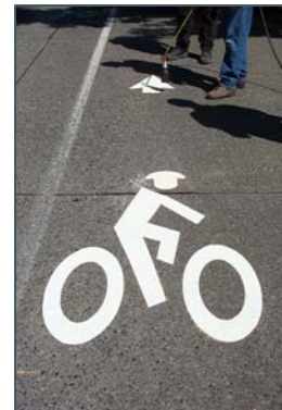
SDOT field crew installs a bicycle lane marking.
