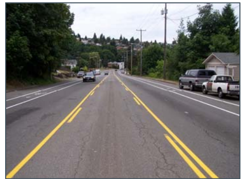
Rainier Avenue S was converted from a four-lane roadway to one travel lane in each direction, a center-turn lane, and bicycle lanes.
