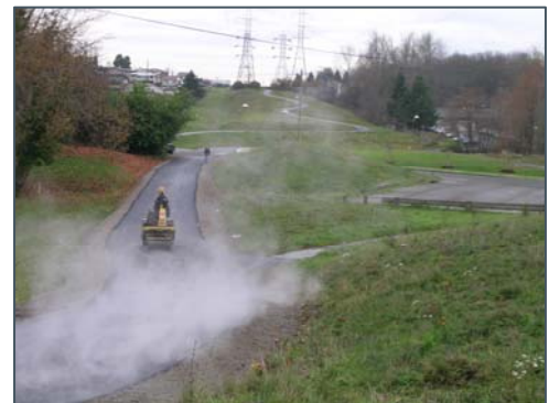
Sections of the Chief Sealth Trail were constructed in December 2006.
