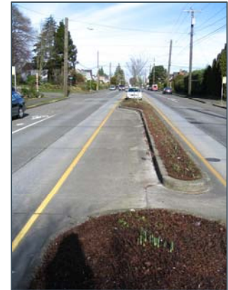
A bicycle-only left-turn pocket has been provided in the median at the intersection of 8 th Avenue NW and NW 77 th Street to help bicyclists cross 8 th Avenue NW.
