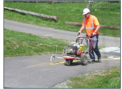
SDOT crew member adds markings at a Chief Sealth Trail crossing.
