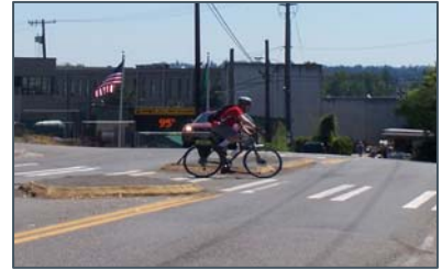
A median crossing island helps bicyclists on the Burke-Gilman Trail cross 30 th Avenue NE.
