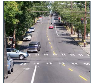
Climbing lanes have been installed on E Union Street to allow slower bicyclists riding uphill to be in a bicycle lane and encourage faster bicyclists riding downhill to move further from parked cars and share the travel lane.
