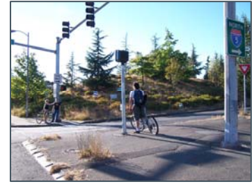
Lack of detection on the street requires bicyclists to cross on the sidewalk.
