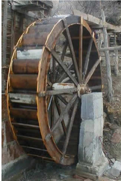
Photograph 3. Montell Seely's Waterwheel in Castledale, Utah (2002).
