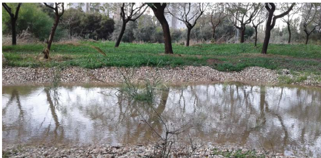
An example of mediterranean rain garden in the city . This garden includes a series of gravel channels and filtration ponds lined with native plants | Photo: Sharon Greenblat
