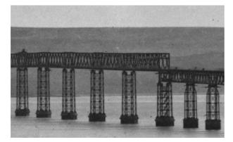
2 Closeup of the join between the high girders at left and the low girders at right on the Dundee side of the bridge. The centre of each high tower shows the diagonal tie bars and horizontal struts which united the two subtowers. Unlike the low tower at extreme right, the tops of the high towers are not reinforced by complete girders
