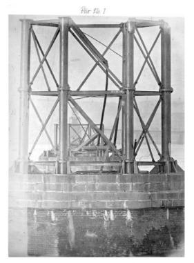
7 Two partly intact tiers on the first pier, photographed from the south looking north. East facing tie bars have all broken on the centre cells, while the west facing tie bars are intact. Breakage has occurred consistently at the lower lugs
