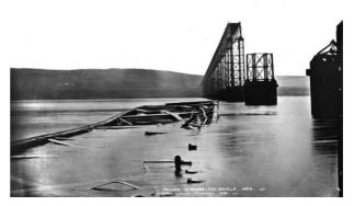
5 Side of the high girders seen at low tide. The girders were found almost intact close to the pier bases, and laid out in a wave form alongside the high section of the bridge
