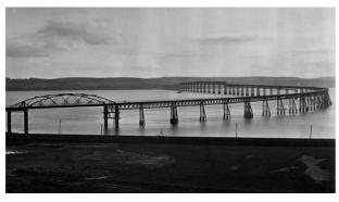
1 The Tay Bridge just after completion, showing the centre or 'high girders' section needed to allow passage of high masted sailing ships upstream along the river to Perth (clearance was about twenty-seven metres at high tide). Some finishing work was still being performed on the bridge, judging by the staging and ladders seen at various points
