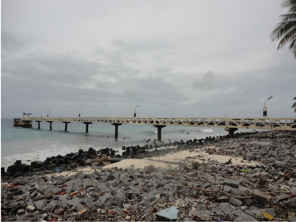
C) Desalination plant-Kavarathi Island
