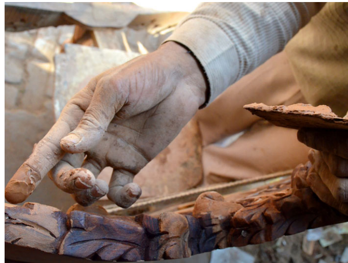
Putty being filled in cracks by the painter.
