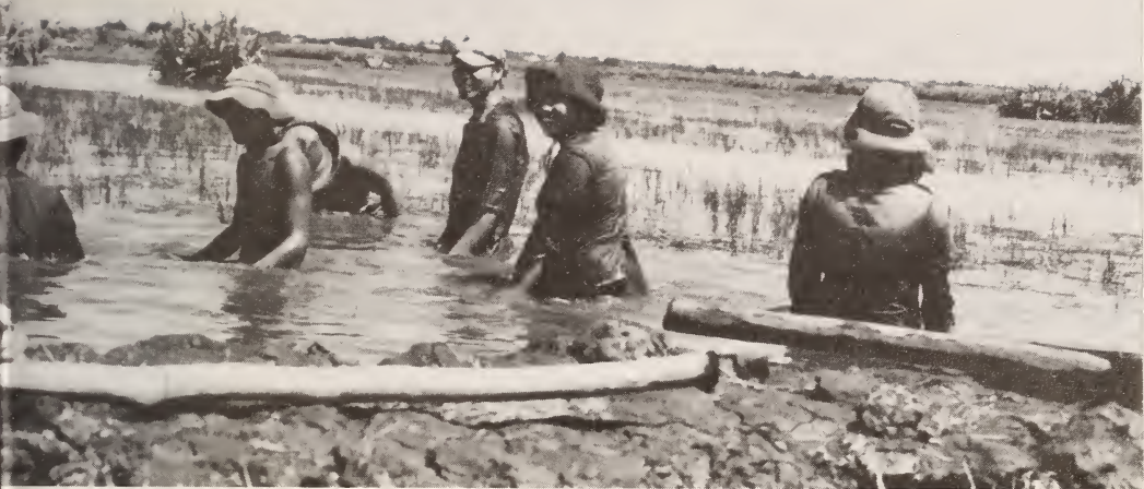
Rice paddy dike construction Courtesy Bill Herod
