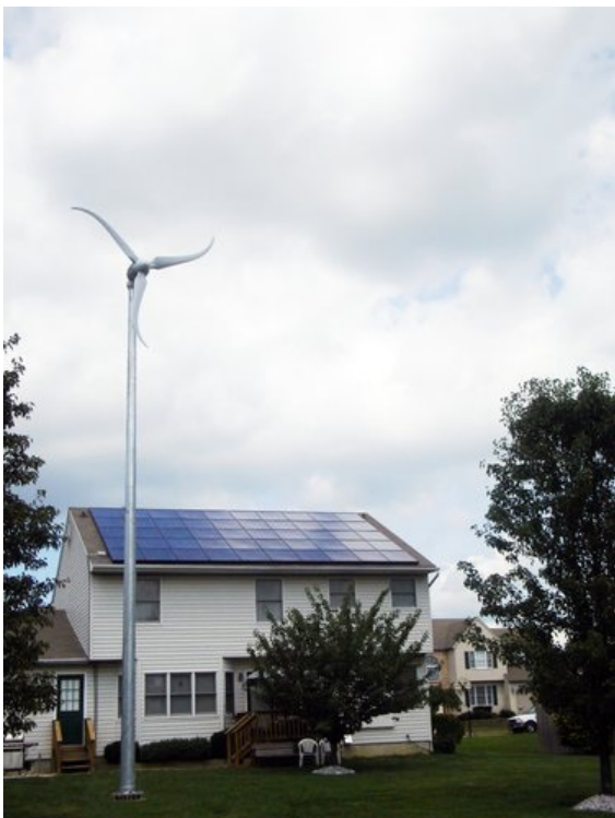
Southwest Windpower's 1.8-kW Skystream wind turbine in a residential application. Photo from Southwest Windpower, NREL 14936
