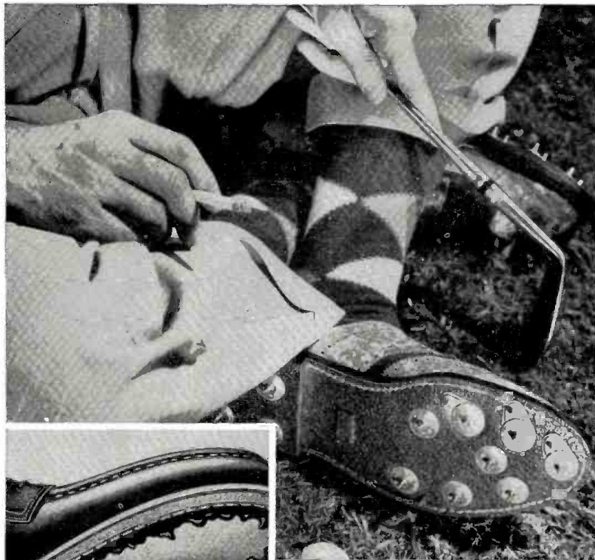
Steel Diet for Golf Shoes. If you play 18 holes of golf on a normal course, you take about 12,000 steps, so a light shoe is very important. The world's largest golf shoe manufacturer found a way to reduce weight by 1/3 - by adding steel construction. The spikes screw into an inner sole plate made from USS Stainless Steel. The resulting shoe is feather-light, flexible as your foot, and you never feel the spikes.
