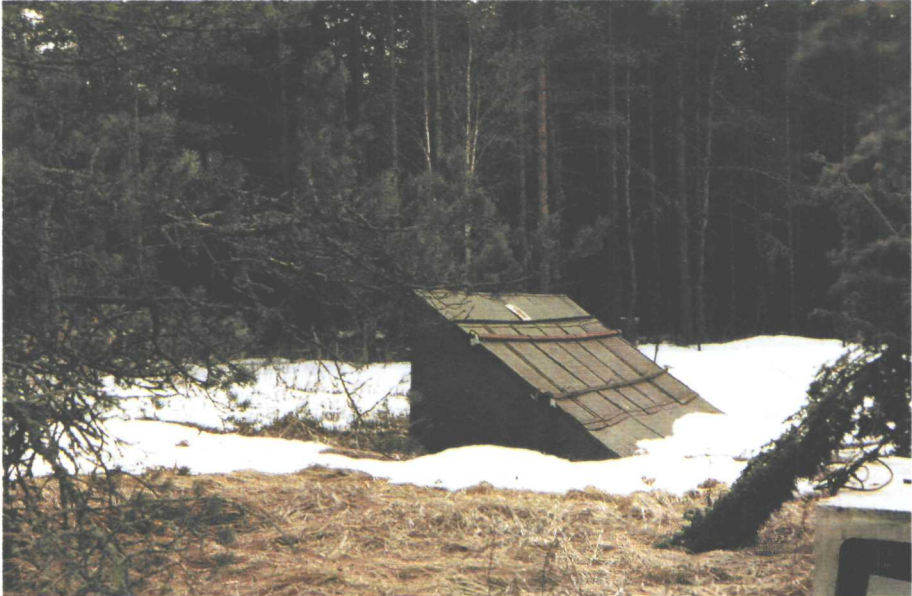
Photo 2. Locked roof cover of the vault.
