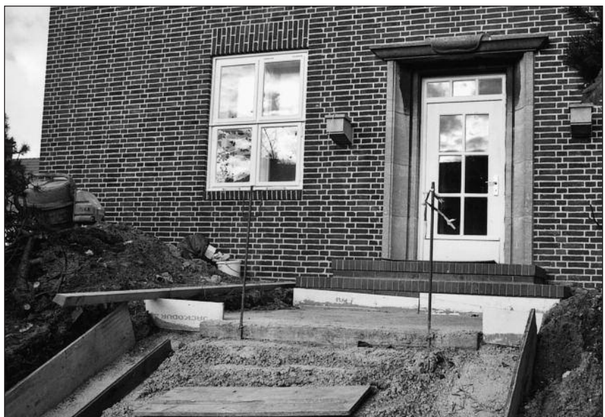
The same building, under repair when we photographed it in October 2004.
