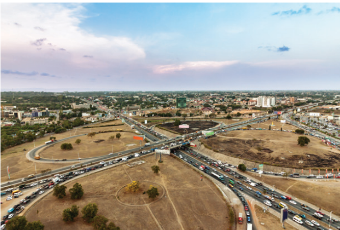
Road infrastructure, Ghana
