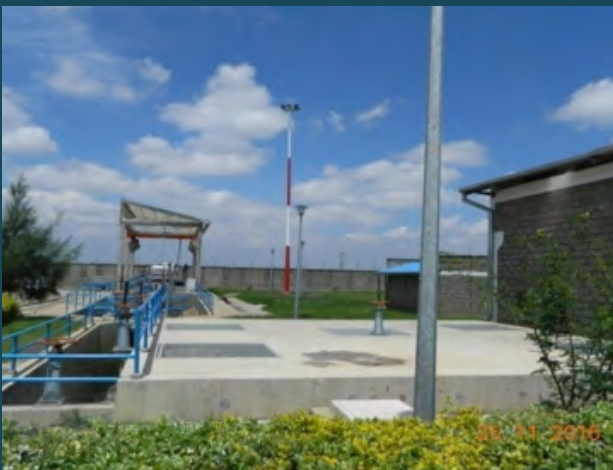
Wastewater treatment plant, Dandora, Kenya
