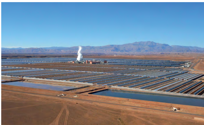
Noor Ouarzazate I (NOORo I) solar power plant, Morocco
