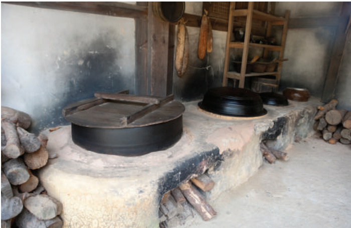
Agungi , or furnace in the kitchen of the Korean traditional house
