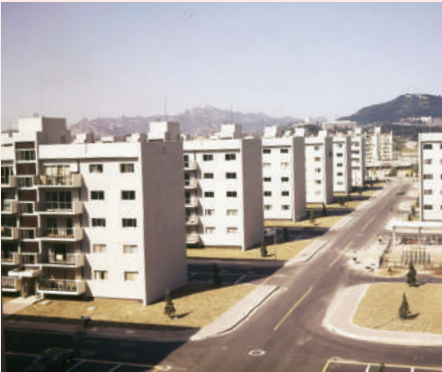
Hangang Mansion Apartment (1970)
