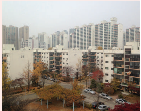
Hangang Mansion Apartment (2016)
