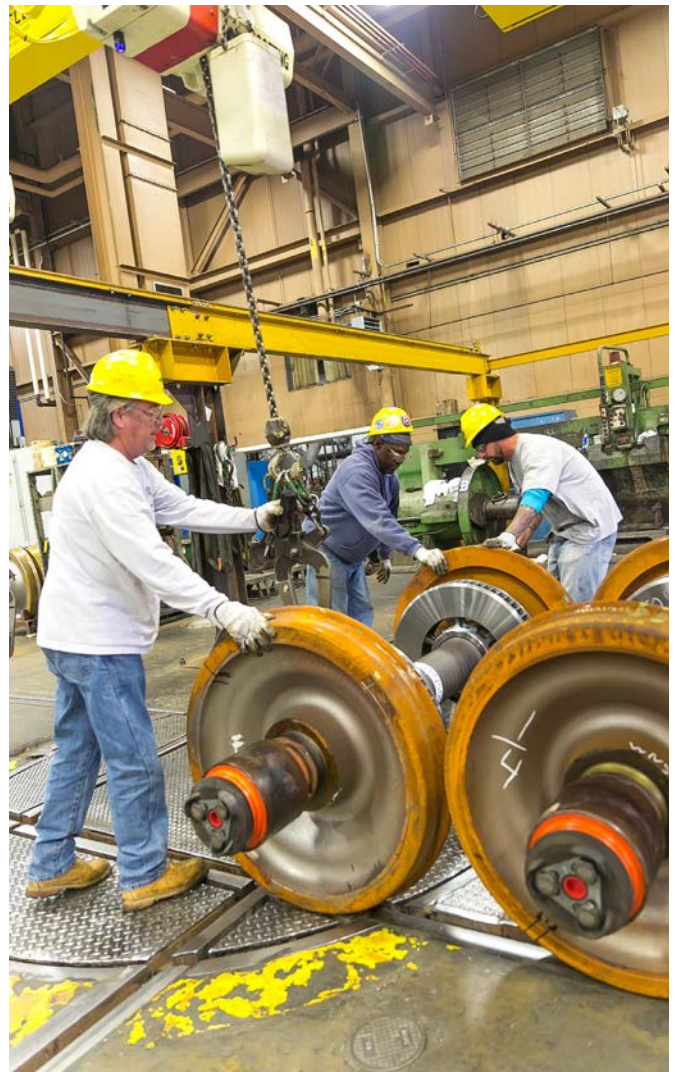
Amtrak staff performing wheel work at the Wilmington Locomotive Back Shop.
