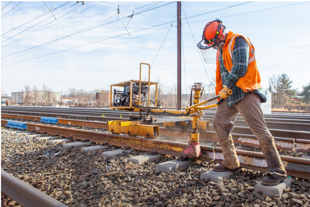
Track Maintenance along the NEC
