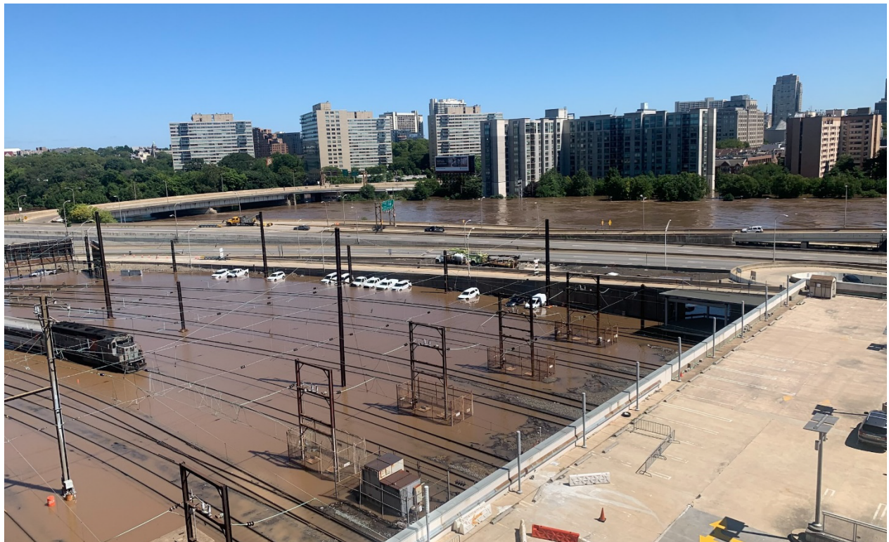
Track Flooding from Hurricane Ida, Penn Coach Yard, Philadelphia, PA
