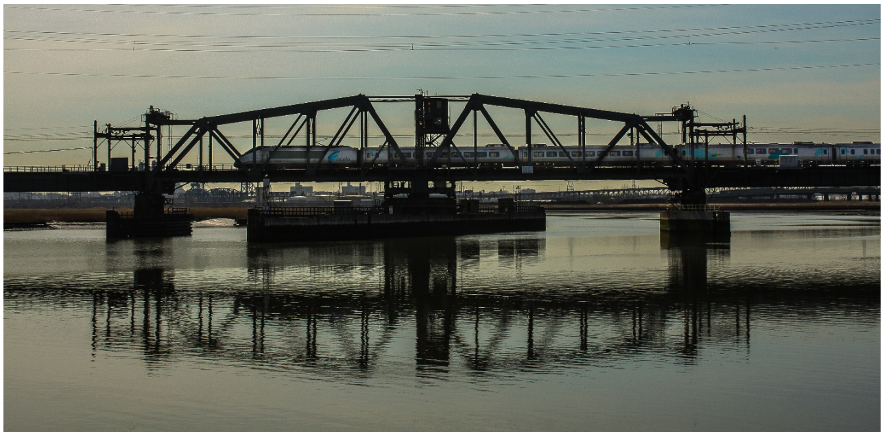
Portal Bridge, New Jersey
