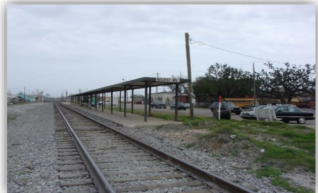
Figure 5: Biloxi, MS Station Canopy
