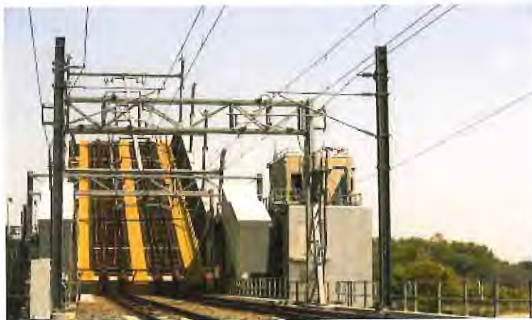
Figure 42. Niantic River Bridge (Amtrak, 2015)
