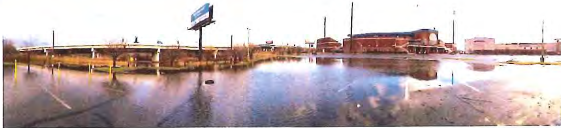
Figure 11. Flooding near Amtrak Training Facility (2009), Wilmington, DE (photo source: Amtrak)
