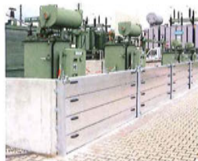
Photo Credit: Flood Control International (floodcontrolinternational.com)
