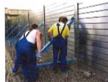
Figure 10. Installation of a Deployable Wall
