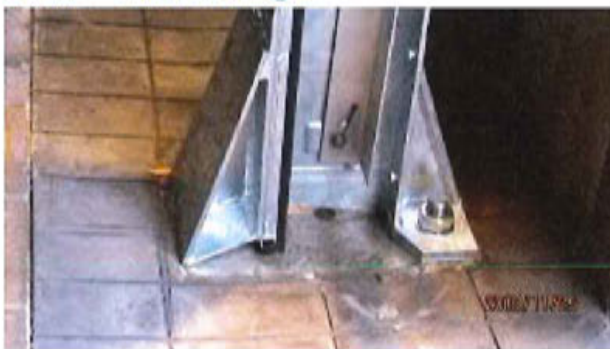
Figure 3. Typical Wall Anchorage System
