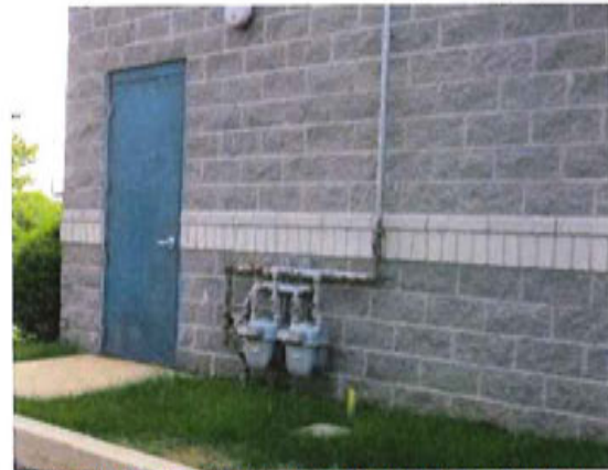
Figure 20. Electric Meter at First Floor at Ground Level
