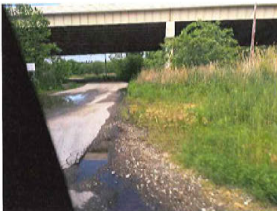
Figure 23. Picture of High Speed Way
