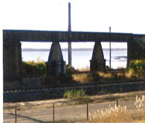
Figure 45. Low Elevation Tracks under Bridge (MP 21.5 to 22.0)
