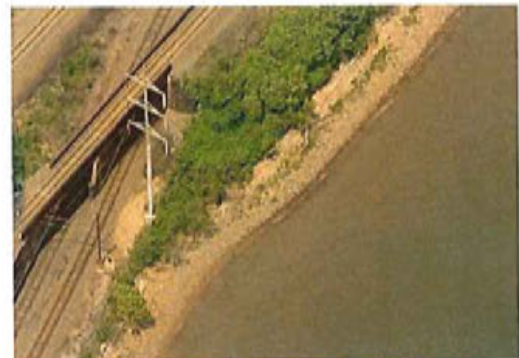
Figure 41. High and Low Elevation Tracks (MP 21.5 to 22.0)
