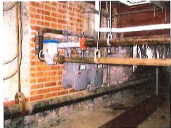
Figure 6. Crawl Space beneath 1st Floor
