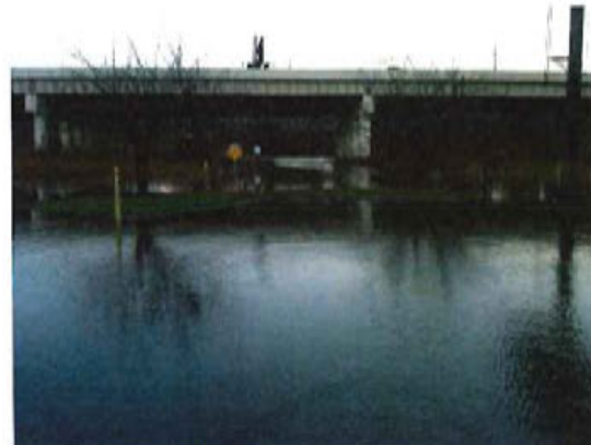
Figure 21. Flood Waters below I-95 Overpass at Access Road Preventing Access to Training Center
