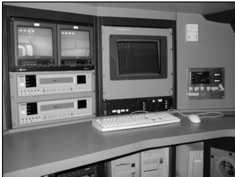
Figure 11. Operator console in Microscale Emissions Modeling System. VCRs and video controls are in the left-hand equipment rack and the PC computer monitor is in the right. AC electrical power system controls and the environmental thermostat are on the far right.
