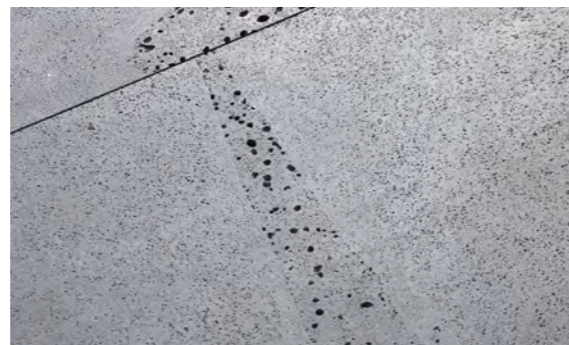
BLUESTONE FEATURE PAVING
