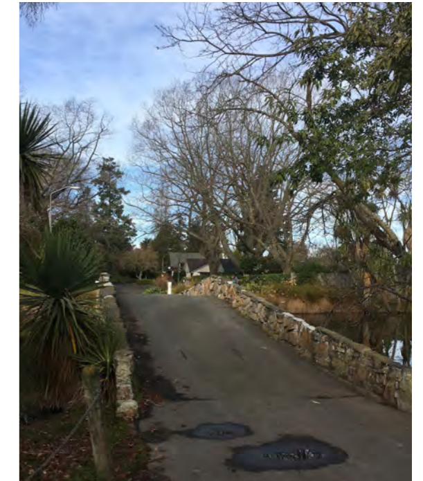
VEHICLE BRIDGE AT CRICKET OVAL
