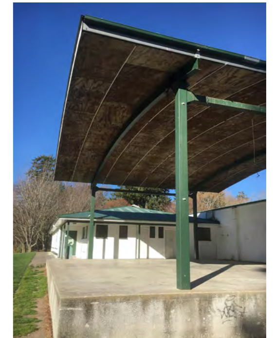
EXISTING COVER OVER PAVILION PERFORMANCE STAGE
