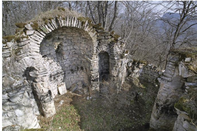
Figure 4 Mokhrenis. Interior view looking NE. Photographs by S. Karapetyan, 2011.
