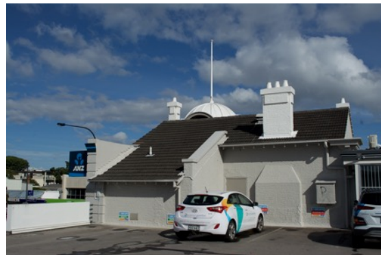
Figure 6: Part of the north elevation viewed from the upper-level carpark, which abuts the rear of the portion of the building (THS, April 2018).
