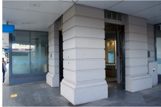
Figure 8: The rusticated base of the clock tower showing the two original entries with fixed top-lights and the partially enclosed verandah along the south elevation (THS, April 2018).
