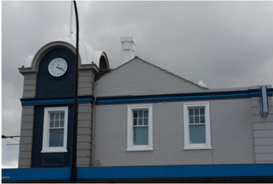
Figure 7: The first-floor of the east (Victoria Avenue) elevation showing the gable roof, dome capped clock tower and timber sash windows (THS, April 2018).
