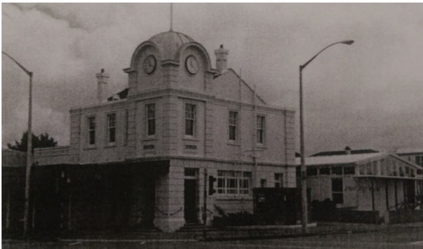
Figure 13: The Remuera Post Office in 1987. Note the small 1936 extension to the left, the 1960s structure to the right and the addition of a verandah to the Remuera Road elevation. It is not known when the latter was incorporated. A new ground floor window was also inserted by this time (H. E. White photograph, from Ivan Clulee, 2011, 13).
