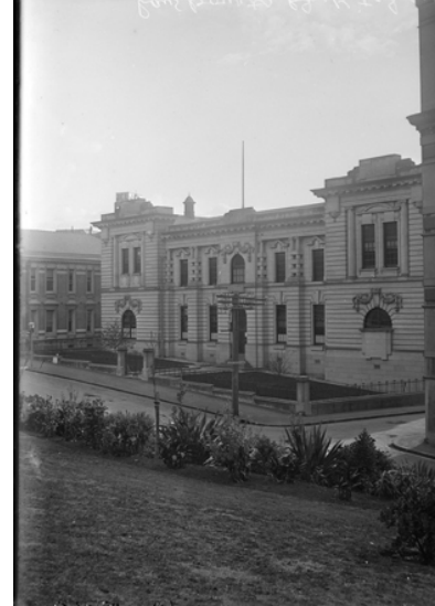
Figure 42: The Magistrates Court, Auckland in 1919 (J. D. Richardson, Sir George Grey Special Collections, Auckland Libraries, 4-1775).
