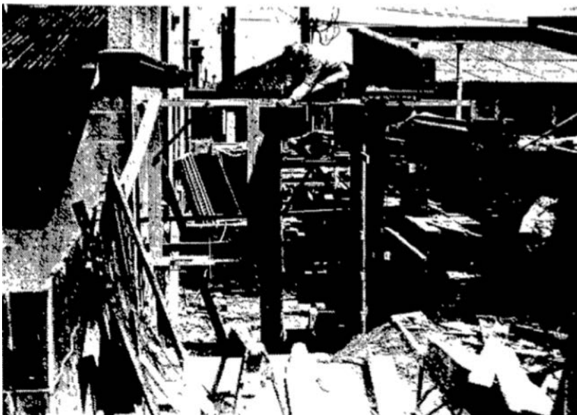
Figure 12: Image published in the Auckland Star , 1936 showing the construction of the Remuera Post Office extension, which was completed in January 1937 (More Accommodation, Auckland Star , Volume LXVII, Issue 281, 26 November 1936, 9, Papers Past).
