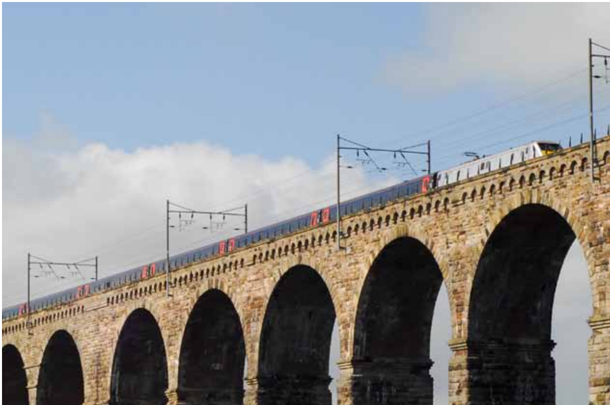
Royal Border Bridge, Berwick-upon-Tweed (Grade II*). OLE installed c. 1989 (photograph: ©flickr.com/photos/forest_pines)
