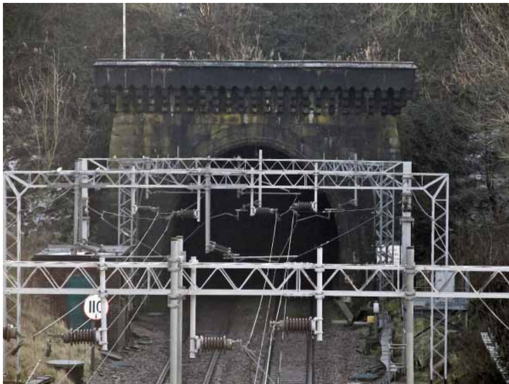
Tunnels: poor practice! Kilsby Tunnel, West Coast Main Line (Grade II*) (photograph: ©Ian Robinson)
