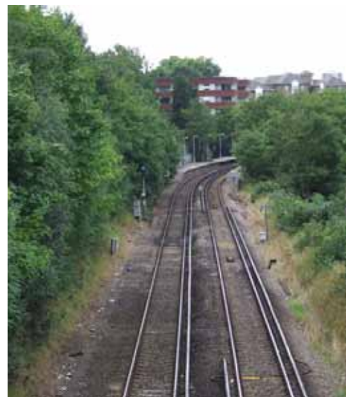
Third rail electrification (photograph: ©Malcolm McDonald)
