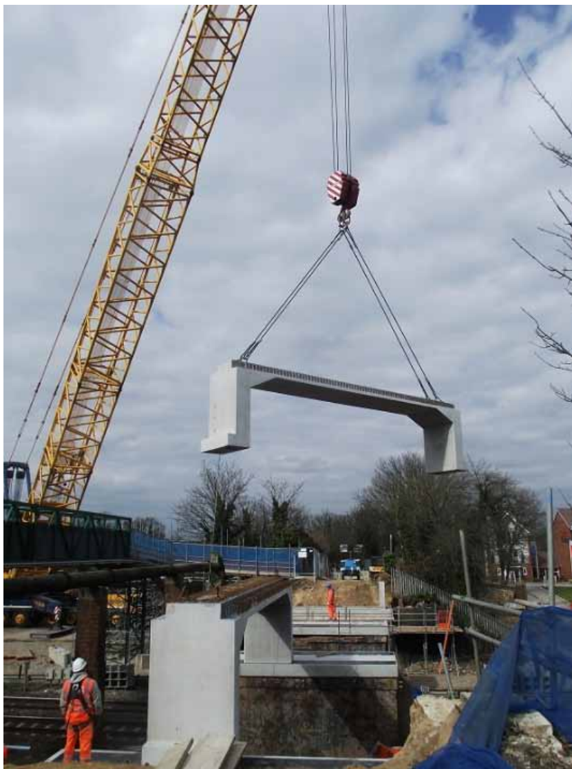
Typical reconstruction of a non-heritage bridge (photograph: ©Network Rail)
