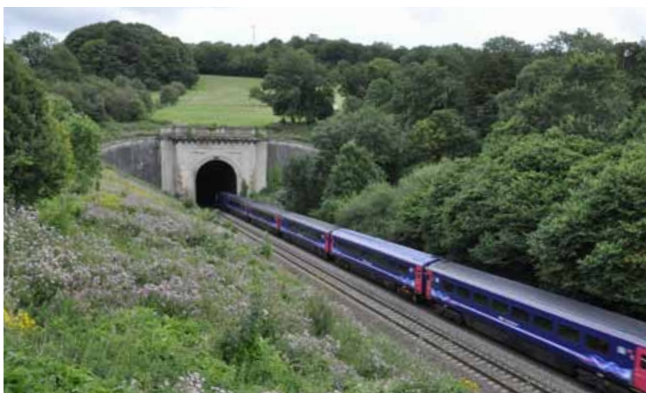
Box Tunnel West Portal, Great Western Main Line (Brunel, Grade I): seen from public viewing area (photograph: ©Alan Baxter & Associates)
