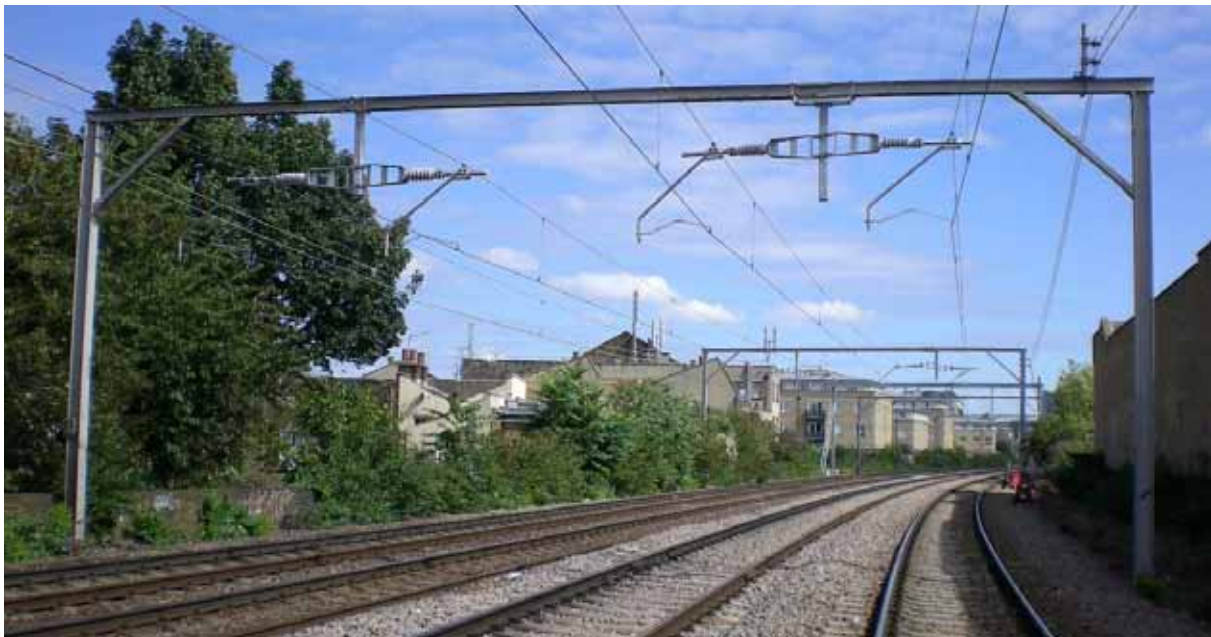
A typical portal frame made of H-section steel members (photograph: ©Network Rail)
