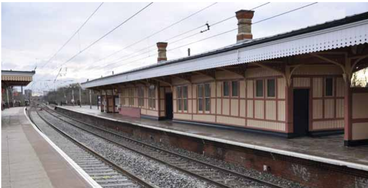
OLE at Hanwell Station on the Great Western Main Line (Grade II). The canopies have been cut back sympathetically (photograph: ©Alan Baxter & Associates)
