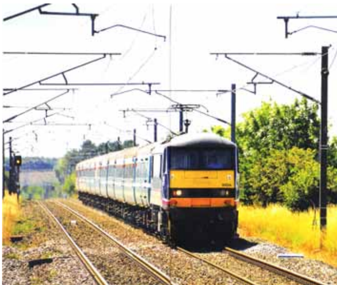
Overhead line electrification (photograph: ©Bill Welsh)
