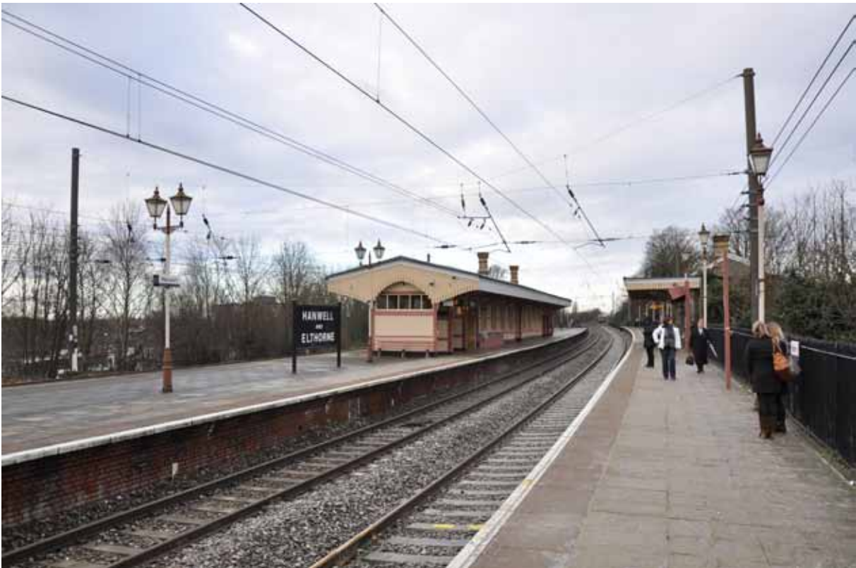
Headspans at Hanwell Station, on the Great Western Main Line. These supports are no longer favoured except where trains move very slowly, such as depots or terminus stations (see section 13.6) [photograph: ©Alan Baxter & Associates]
