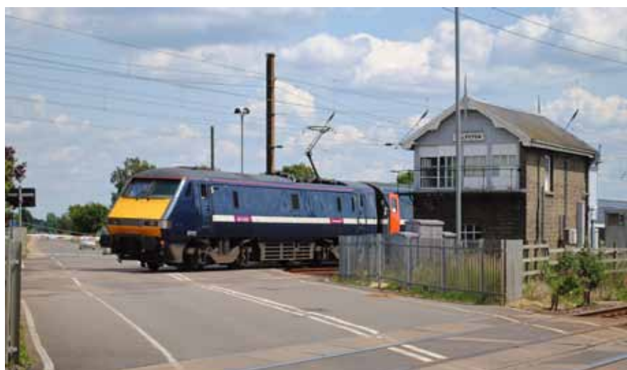
Level crossings - note how the pantograph on the train is extended to reach the raised contact wire [photograph: ©Philip Hilbert]
