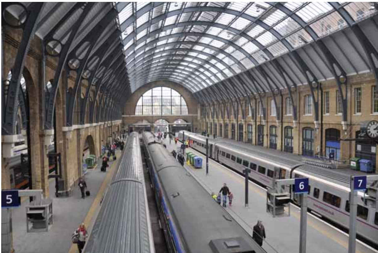
OLE inside Kings' Cross Station, 'camouflaged' by the backdrop of the trainsheds (photograph: ©Alan Baxter & Associates)
