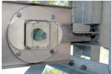
Disconnecting circuit breaker unblocked in open position.
