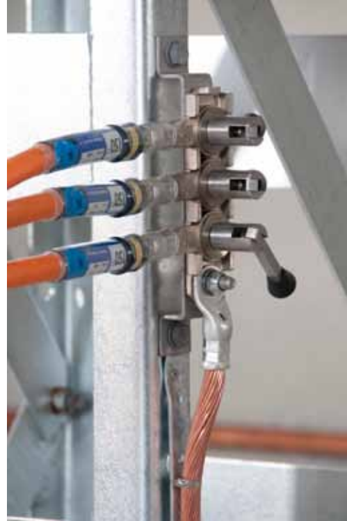
Connection clamp for earth connection
