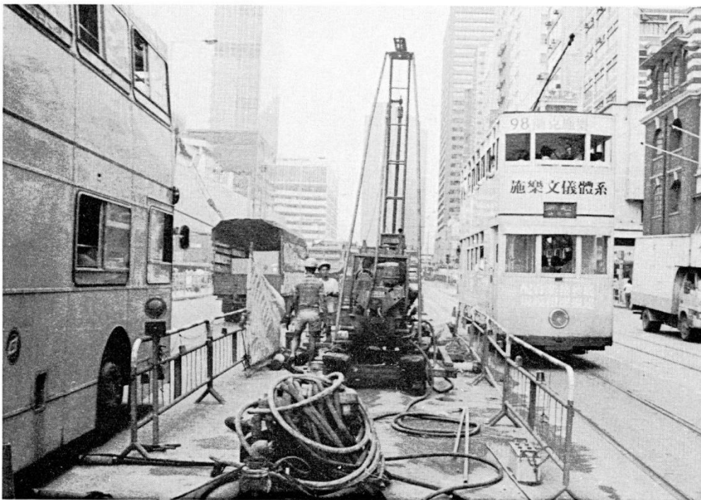
B : Drilling in the Middle of a Busy Road
