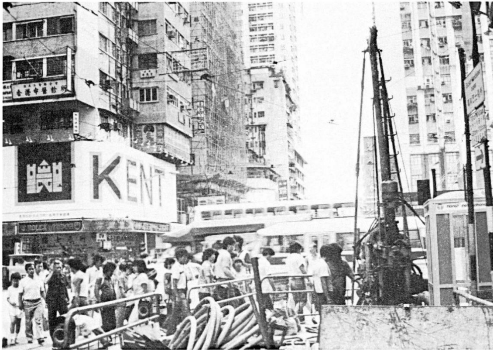
A : Drilling in a Densely - developed Urban Area
