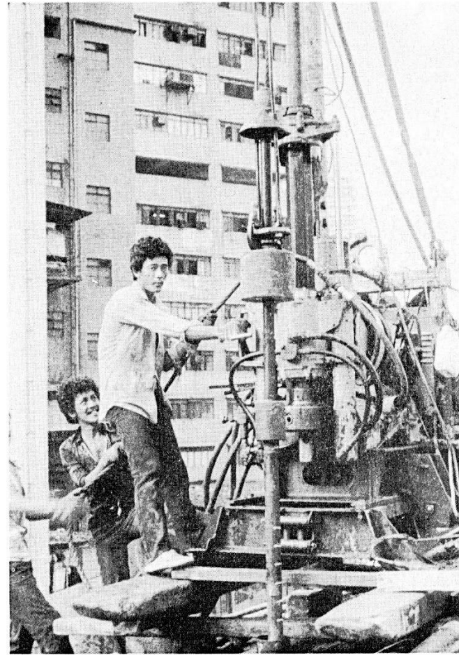
B : Automatic Release Trip Hammer and Drill Rods
