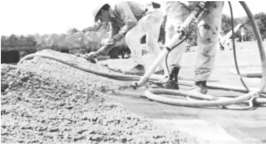
Figure 22. One worker applies portland cement plaster to an amusement park structure while another (background) floats the plaster and embeds the mesh. (30570-M)
