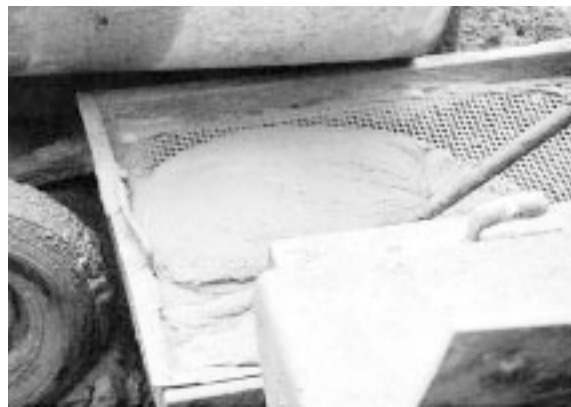
Figure 14. Step 4) Last, add the balance of the sand and water required to achieve desired consistency. Mix from 3 to 5 minutes. (66134)
