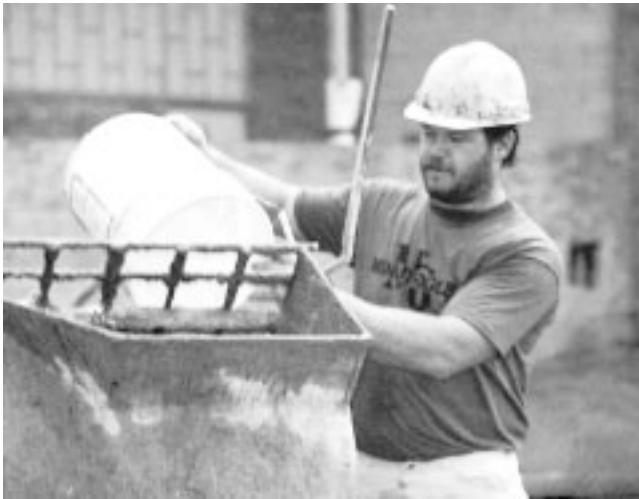
Figure 11. Step 1) Place water in mixer first. (66131)
