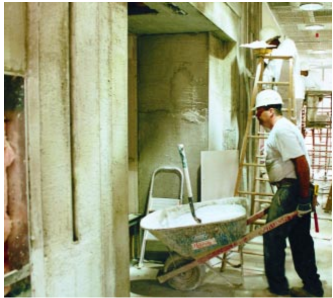
Figure 16. On this job, plaster was distributed by wheelbarrow to mortarboards. (IMG12627)
