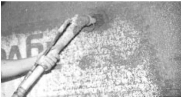
Figure 22. One worker applies portland cement plaster to an amusement park structure while another (background) floats the plaster and embeds the mesh. (30570-M)
