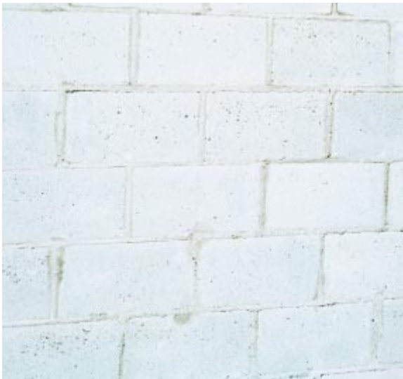
Figure 7. Joints on concrete masonry to receive plaster are struck flush. (66130)
