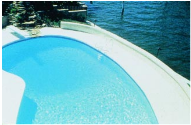
Figure 26. White portland cement plaster is an attractive and durable interior finish for swimming pools. (52983)
