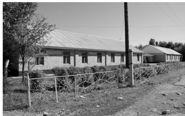
Fig. 5 11 years course school in Kaipov village.
