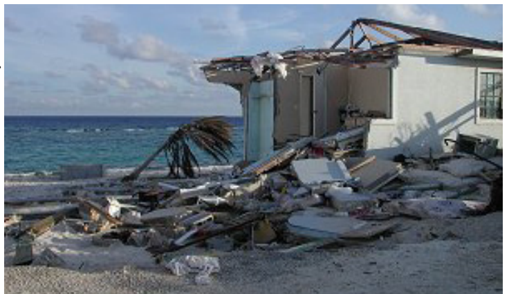
Damage from Hurricane Ivan
