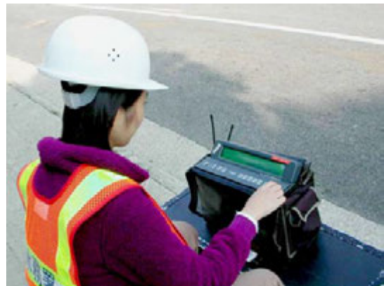
Plate H8 Leak Pinpointing by Leak Noise Correlator
