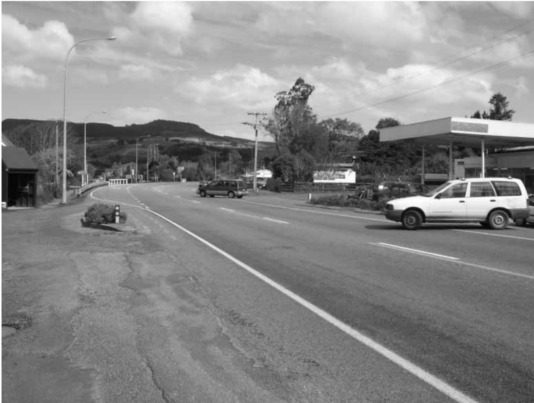
Figure 3-1 : SH1 at the Blueskin General Store. Taken from opposite the Store at the bus stop looking to the south. Note the two vehicles exiting from the Blueskin General Store accesses.
