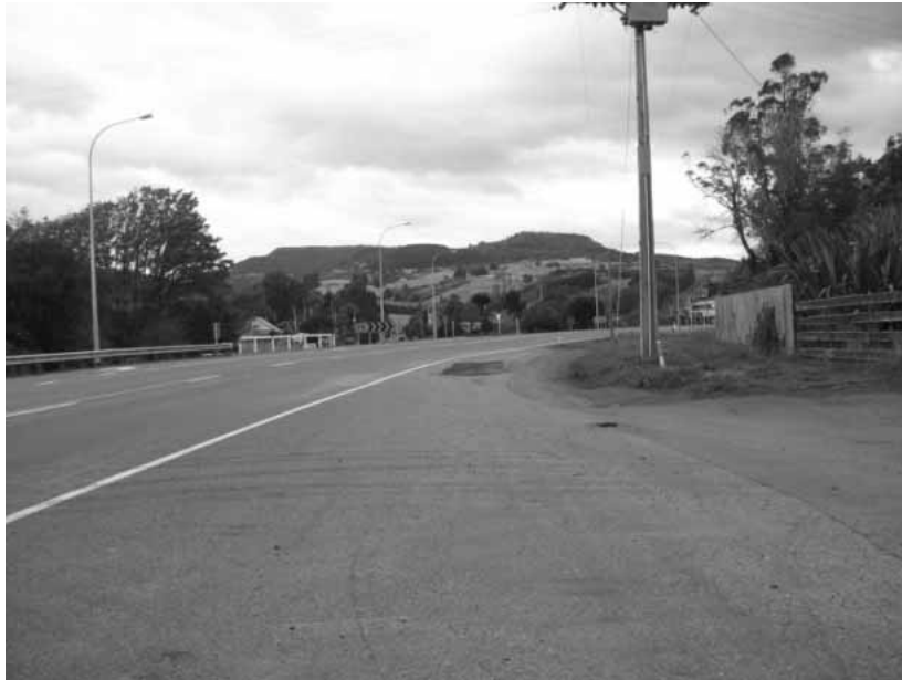
Figure 3-2: View from Blueskin General Store Access to South
