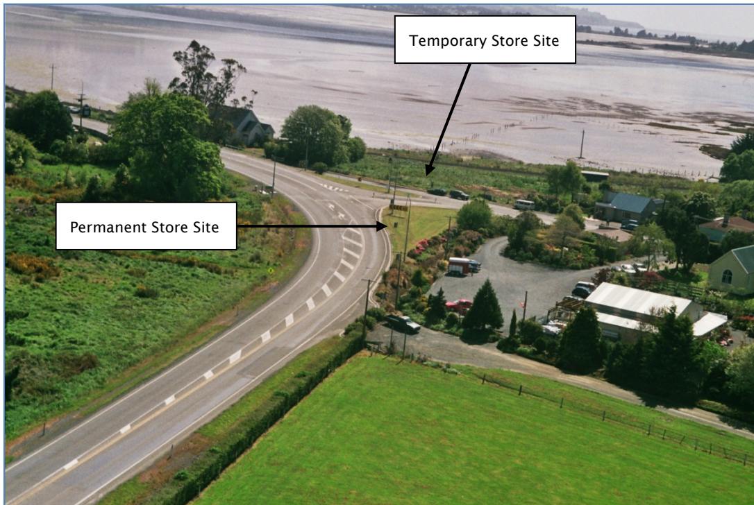
Figure 2-2 : Looking north along SH1 at the Harvey Street intersection. The temporary building will be to the north of Harvey Street. Blueskin Nursery and Cafe is centre right and Blueskin Bay is in the distance.
