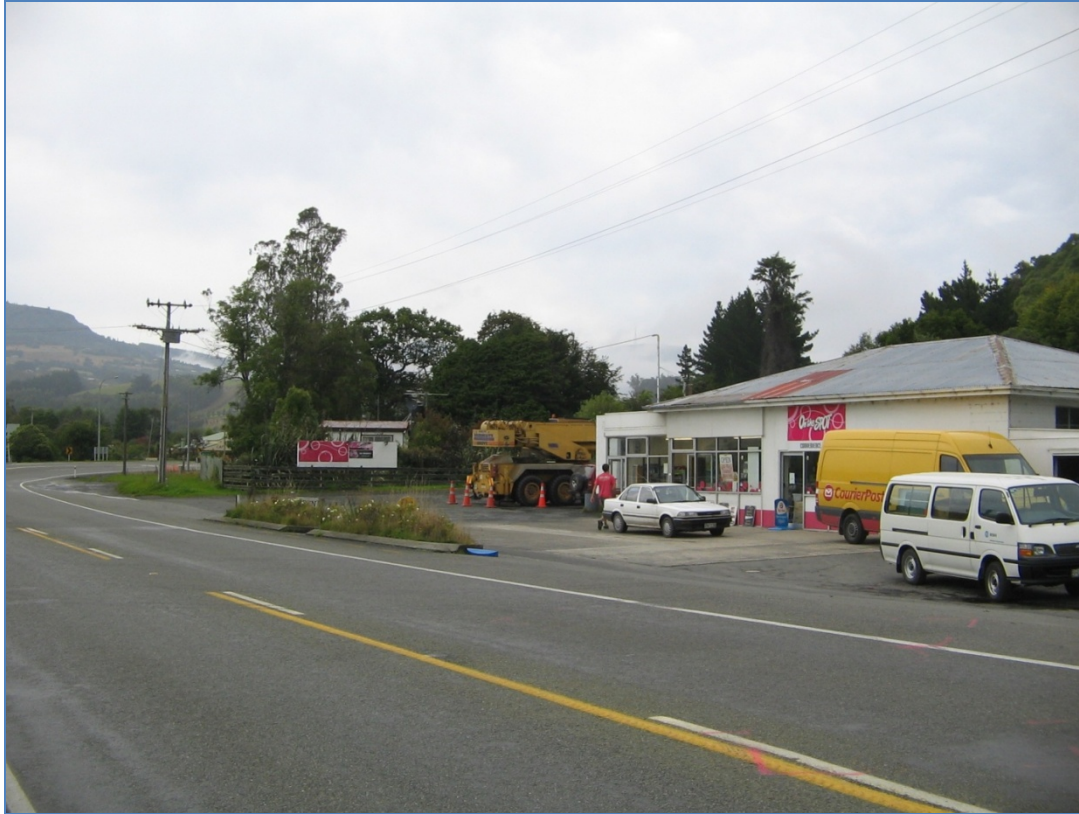
Figure 4-1 : Looking south at the Existing Blueskin Store and parking, on SH1.
