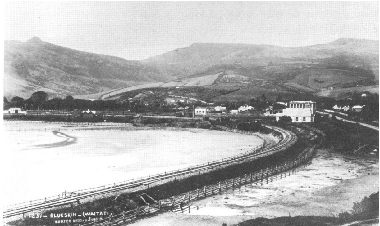
Historical view south towards Waitati from vicinity of Double Hill Rd showing rail line with stone culvert and post-and-rail fences along either side of embankment (Burton Brothers photograph, Hocken Collections E1173/6). Note mudflat on both sides of rail line.
