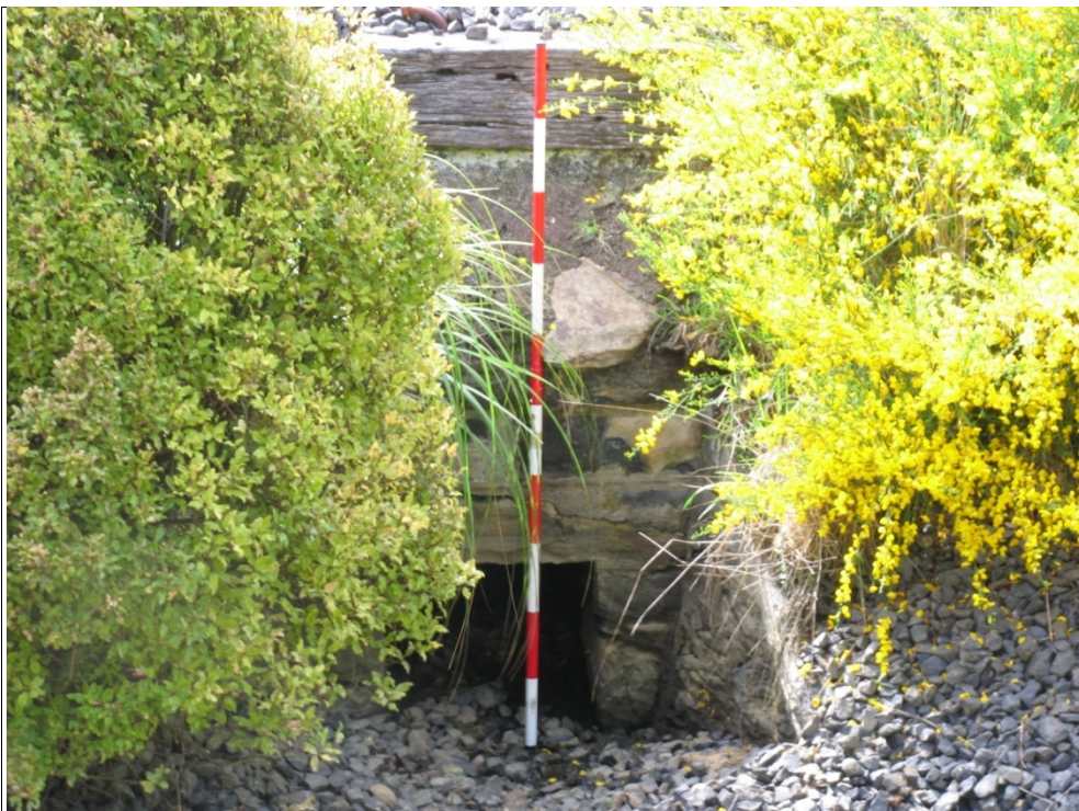
Figure 11. Stone culvert under railway embankment.
