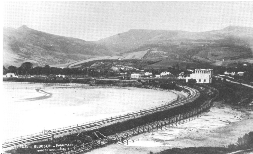
Figure 12. Historical view south towards Waitati from vicinity of Double Hill Rd showing rail line with stone culvert and post-and-rail fences along either side of embankment (Burton Brothers photograph, Hocken Collections E1173/6). Note mudflat on both sides of rail line and culvert in foreground.
