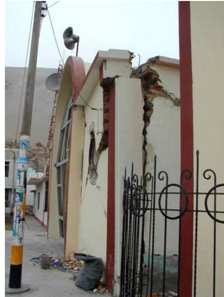
Figures 30 and 31. Church in Ocoña built using very poor construction materials; both the mortar and brick were weak. Previously damaged and patched following earthquake 4 years ago. (Photos by E. Fierro)
