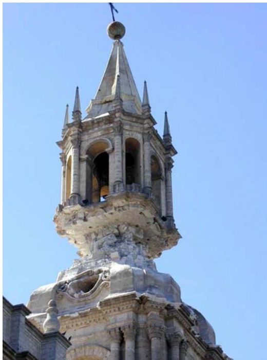
Figures 12 and 13. The precarious tower is supported by four 35 cm by 35 cm concrete columns and four steel rails. One of the steel rails buckled. Arches attached to the main structure were also damaged. (Photos by E. Fierro)
