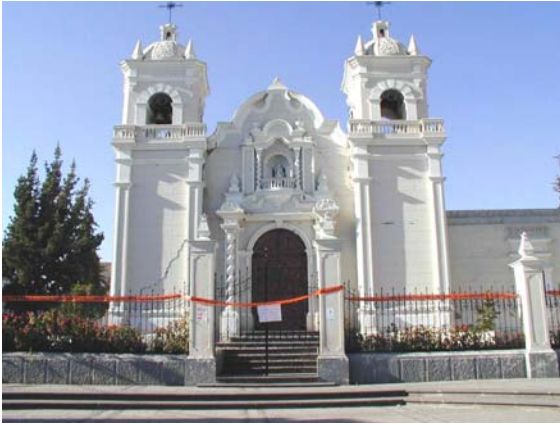
Figures 14 and 15. Church of Santa Marta; towers pulled away from the main structure. Buttresses supporting the main structure show signs of distress. (Photos by E. Fierro)
