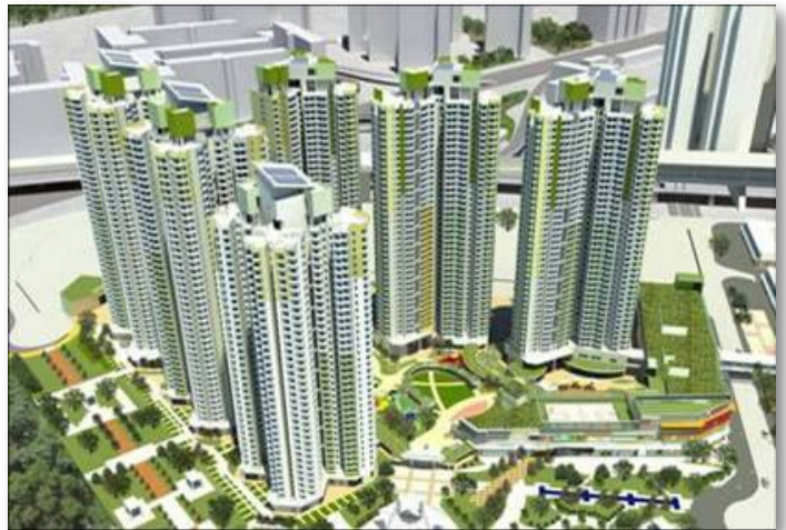
Kai Tak Site 1A project design with the application of Carbon Emission Estimation method to benchmark the carbon emission levels throughout the project life cycle
