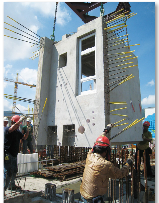
Volumetric precast bathroom in Kai Tak Site 1B
