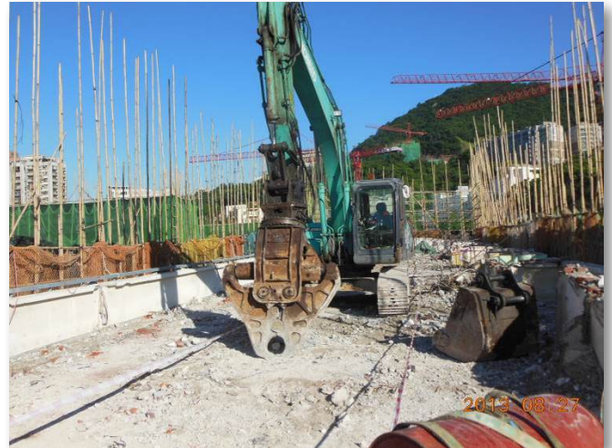
Employing hydraulic concrete crusher at site
