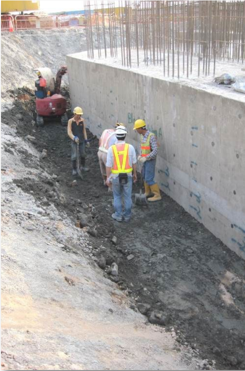
Use of cement-stabilised marine mud for backfilling
