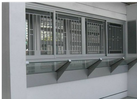
Acoustic balconies and architectural fins
