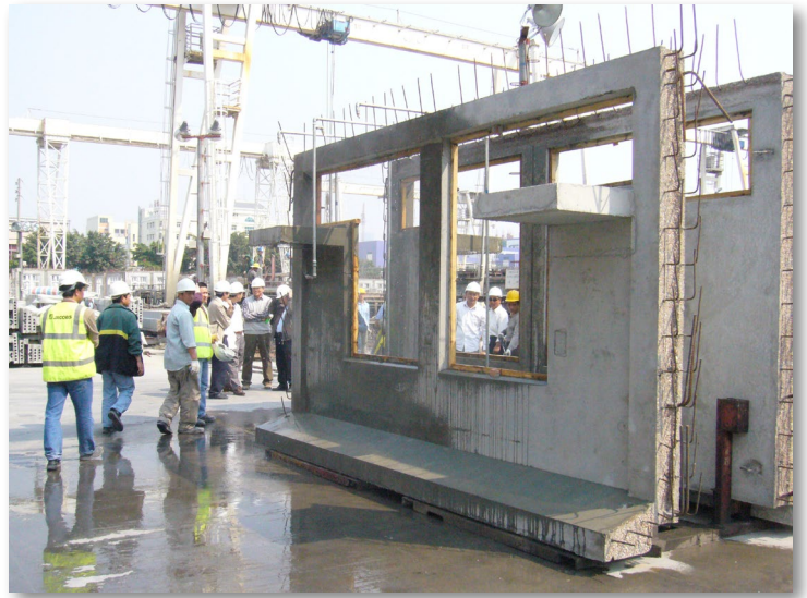
GGBS as a partial substitute of cement in precast concrete facades
