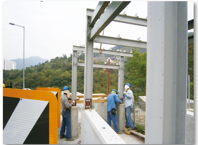
Re-usable modular hoarding at Anderson Road Sites
