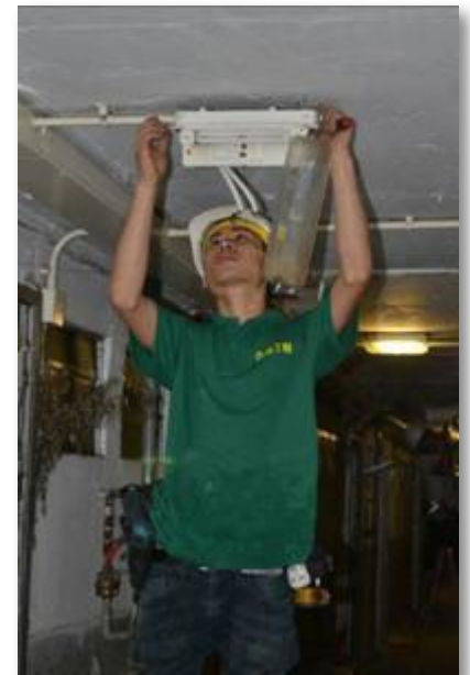
Installation of energy-saving electronic ballasts
