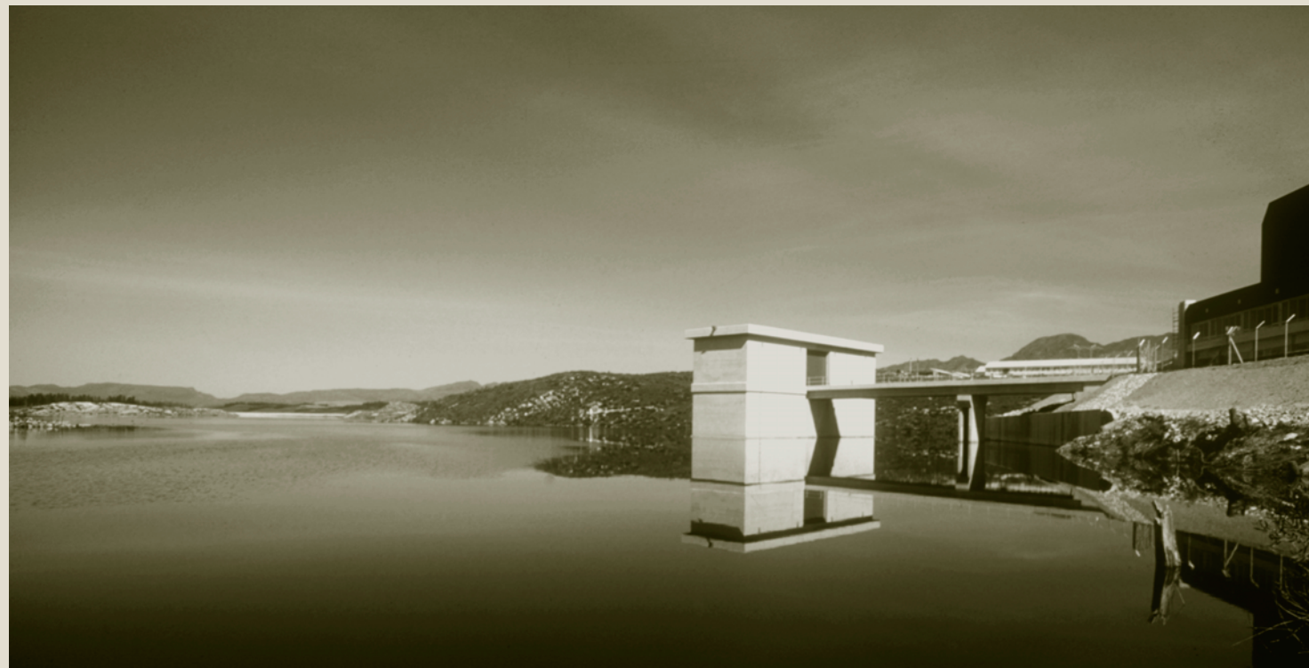
THE TAILRACE STRUCTURE IN KOGELBERG DAM
