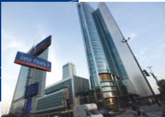
Frontex headquarters, Warsaw
