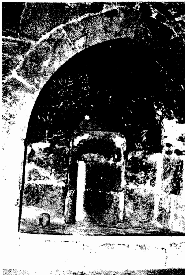
In 1216 the defences of Ajlun castle were greatly strengthened. Many of the new chambers had arrow-slits in rectangular recesses big enough to house a ziyar or frame-mounted crossbow.
