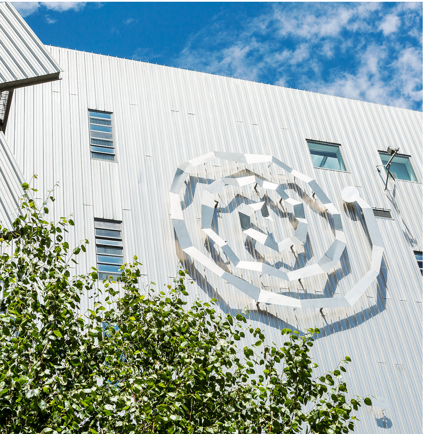
Back of Ben Pimlott Building
