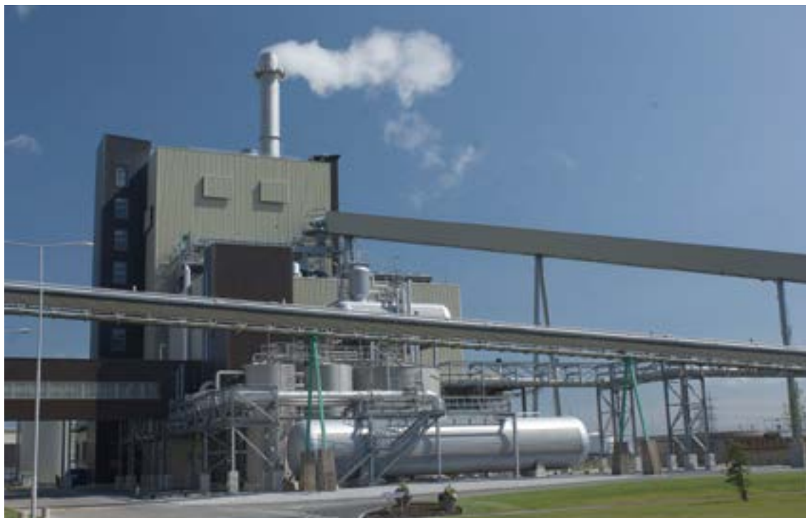
UPM Shotton Paper Mill Renewable CHP (Courtesy of UPM)
